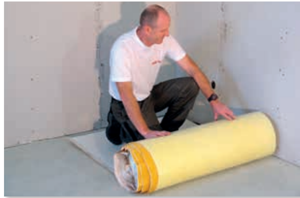
Un-wind the layer on the floor (logos on top)
