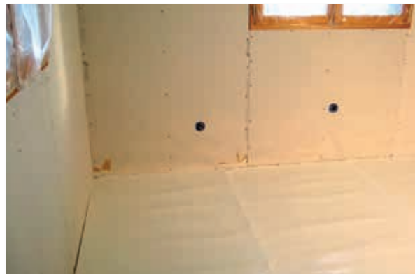
Cover the entire surface
