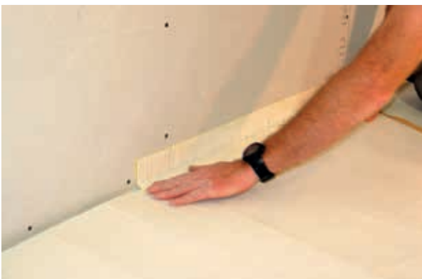
Cover the bottom part of the walls
