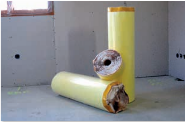
Separate the rolls to apply in a clean surface area
