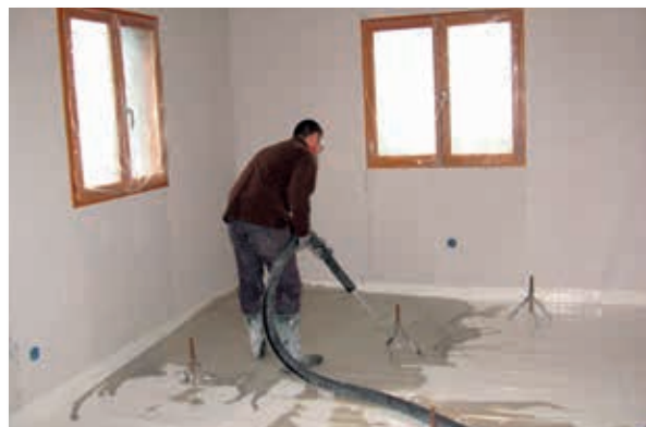
Apply the floating floor
